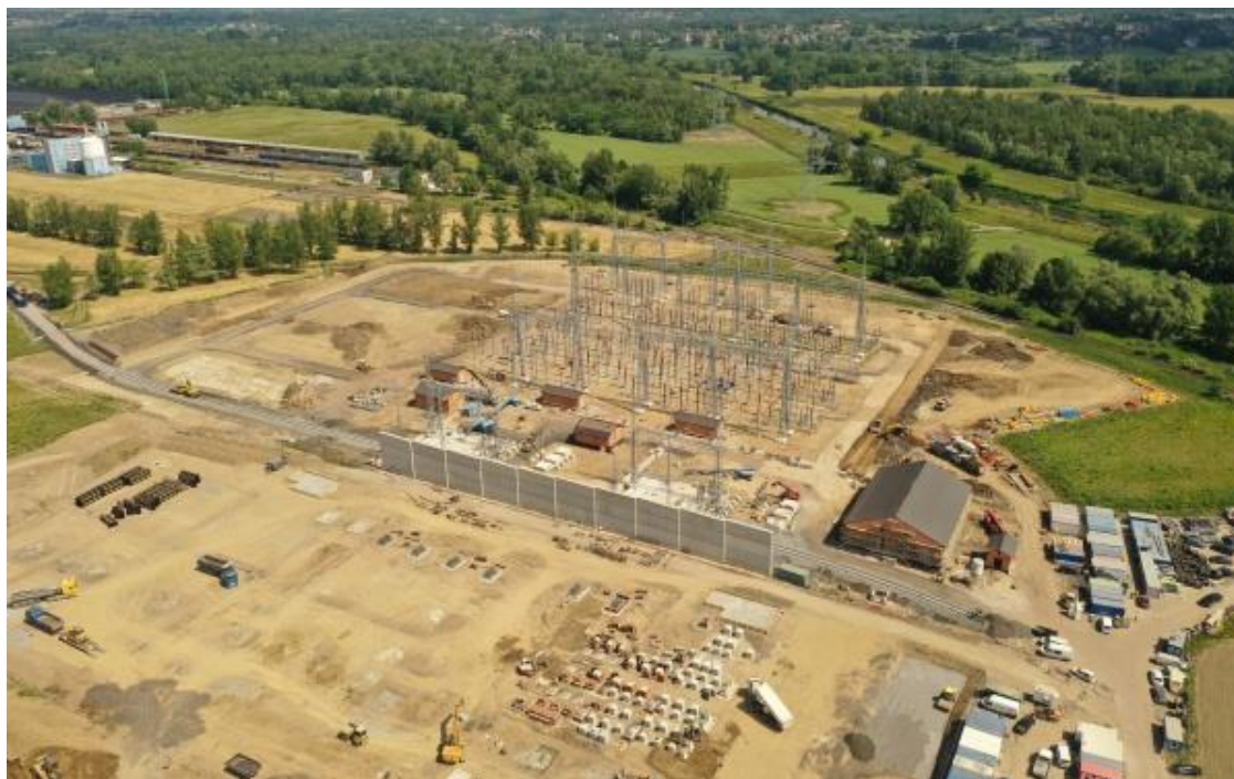
Fig. Construction of a new transformer station in Dětmarovice, Czechia
